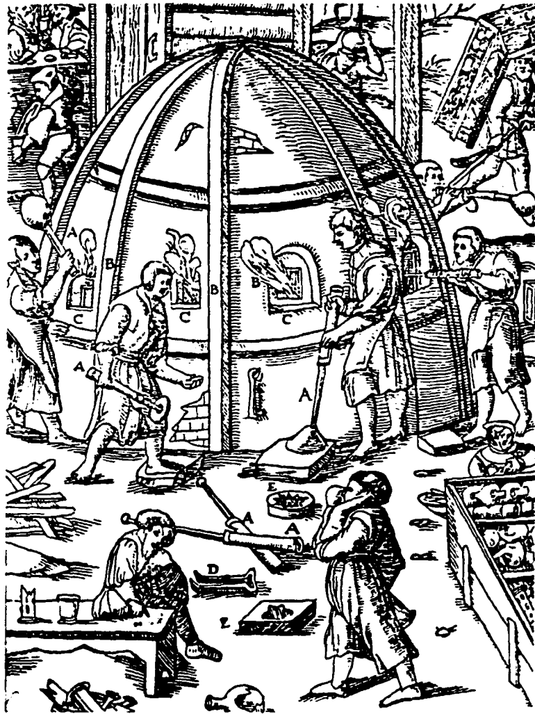
Fig. 8.5. Primary furnace from Agricola's manuscript
